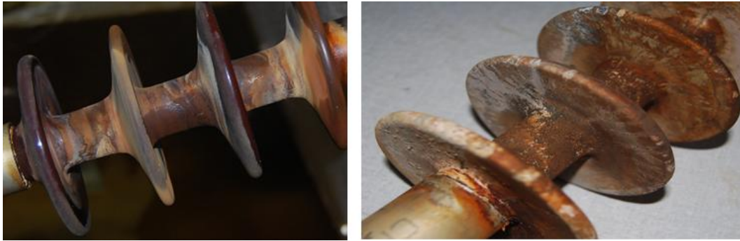
Figure 4.86: Channel 5 and Channel 6 after the test with negative polarity HVDC excitation
