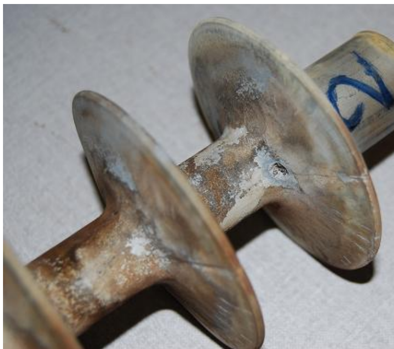
Figure 4.50: Detailed view of aging of the HTV SR insulator (Channel 2) for positive polarity HVDC excitation
