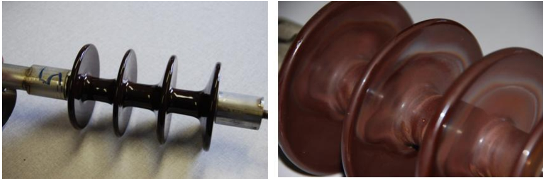
Figure 4.35: Reference porcelain insulator (Channel 5) before and after the test for HVAC excitation
