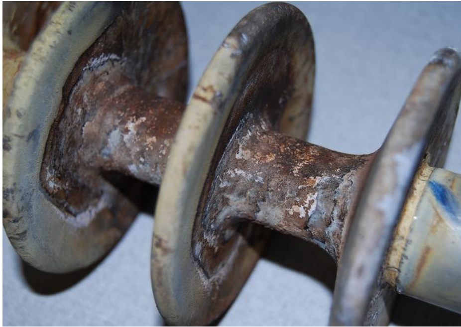
Figure 4.61: Detailed view of aging of the RTV SR coated porcelain insulator (Channel 6) for positive polarity HVDC excitation
