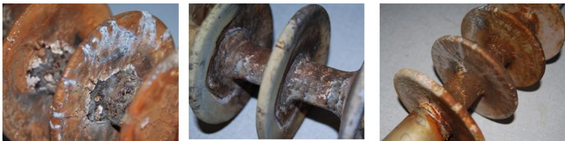
Figure 5.26: Comparison of material aging of the RTV SR coated porcelain insulator (channel 6) for HVAC and positive and negative polarity HVDC excitation
