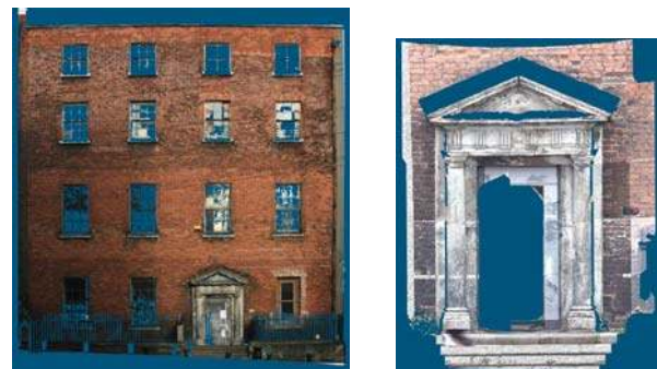
Figure 12. Ortho Imagery from Laser Scan Survey.
