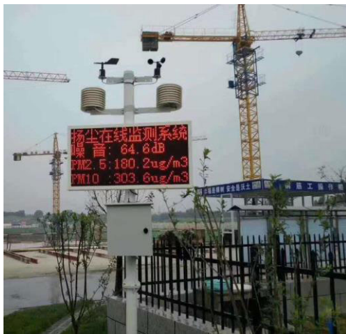
FIGURE 10. Environmental monitoring system of the construction site.
