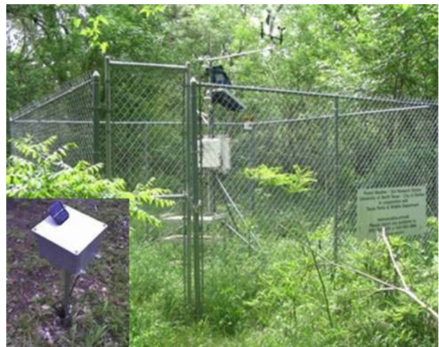
Fig. 8 The GBC weather station and the weatherproof installation box for motes
