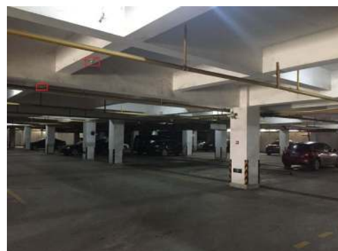
FIGURE 13. Underground parking lot.
