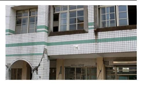
Fig. 5 The device is inspecting the damage on a first floor column
