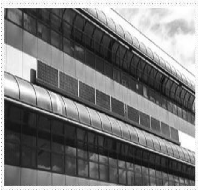
Figure 5: Technology Center PV System
