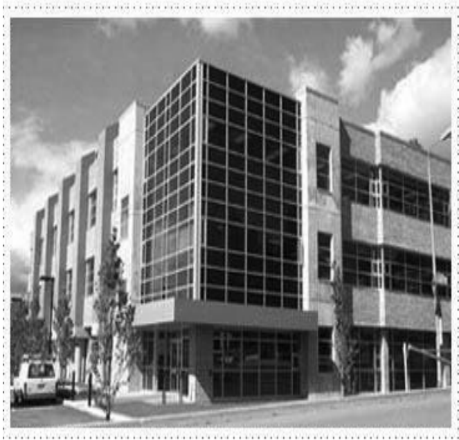
Figure 4: Technology Place PV System
