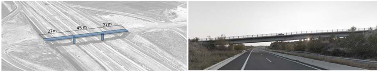
Figure 2. General overview of the bridge configuration.
