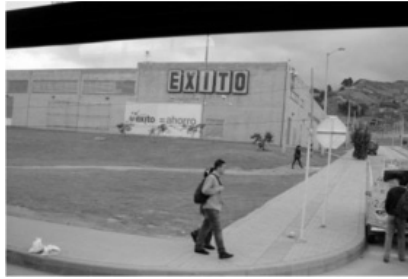
Figure 5. Terminal Suba—sidewalk with good pavement, but without access for people with reduced mobility
