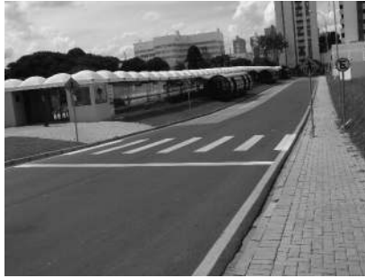
Figure 7. Terminal Cabral, Curitiba—sidewalk with good pavement, but without access for people with reduced mobility
