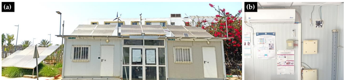
Figure 1. (a) Energy Efficient Building Lab (EEBLab) test site; (b) Interior side wall of EEBLab with ventilation fan and a set of sensors and other equipment.
