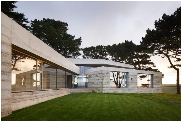
Figure 13: Exposed hand-crafted concrete done horizontally (Frearson, peter-zumthor, 2018)
