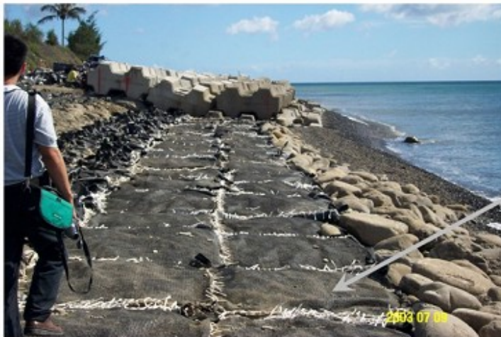
Fig. 1 Geogrid containers used in a pilot test on seashore protection. (Huang and Liao, 2007)
