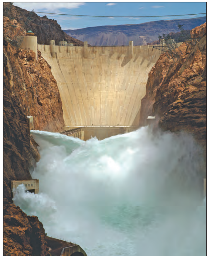
Jet flow gate testing at Hoover Dam, June 1998. Photograph by Bureau of Reclamation.
