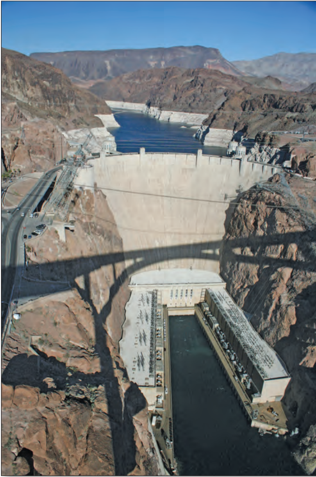
View of Hoover Dam from the new Mike O'Callaghan–Pat Tillman Memorial Bridge (Colorado River Bridge). Photograph by Michael R. Rosen, U.S. Geological Survey.
