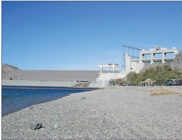
Davis Dam, near Bullhead City, Ariz., which created Lake Mohave, rises approximately 140 ft (42.7 m) above the level of the Colorado River. It is a zoned earthfill structure with concrete spillway, intake structure, and power plant. Photograph by Michael R. Rosen, U.S. Geological Survey.
