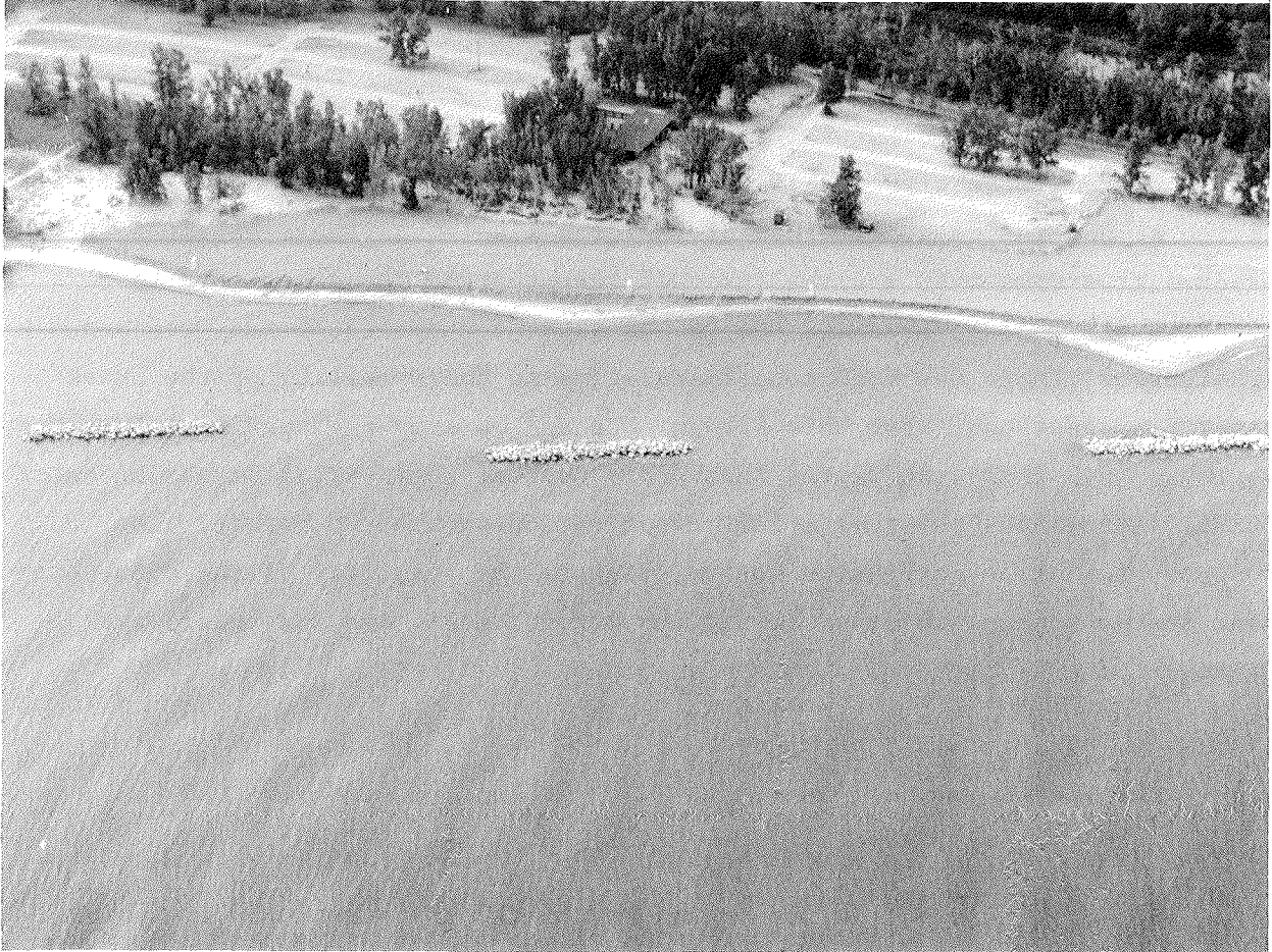
Figure 2. Existing breakwaters at Presque Isle Peninsula
