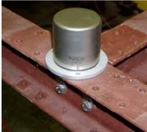
Figure 13. Plate removal at N3 for DC2
