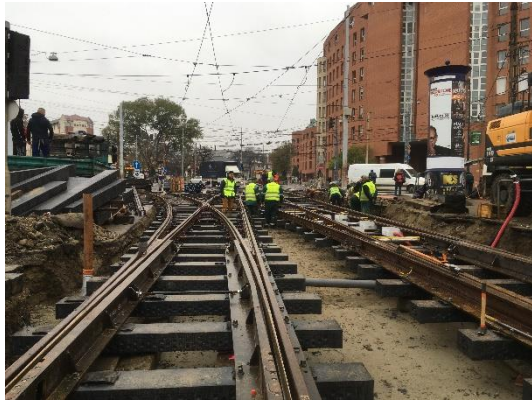
Fig. 4. Concreted ballasted track superstructure during construction
