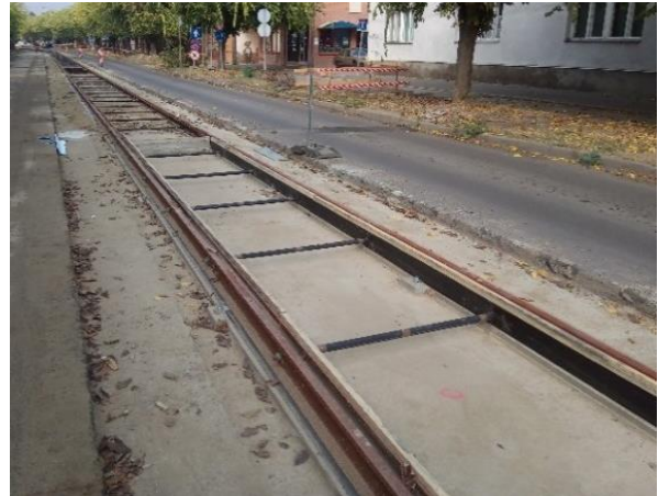
Fig. 8. ESCR B I. track system during construction
