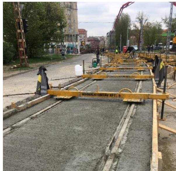
Fig. 10. ESCR B II. track system during construction
