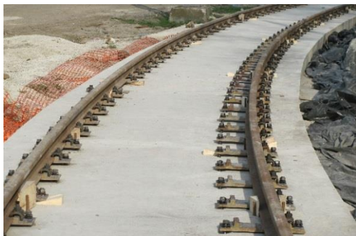
Fig. 6. Concrete slab track during construction
