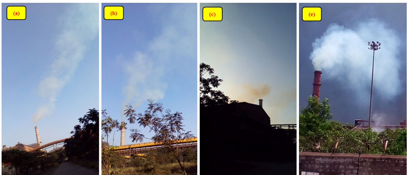
Fig. 3 Stack emissions a, b reddish and whitish appearance, afternoon hours, c reddish appearance, evening hours, as seen from the east side, d whitish appearance in a cloudy weather (Color figure online)
