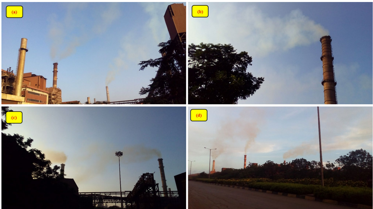
Fig. 2 Stack emissions a afternoon hours, reddish and yellowish appearance, b reddish, whitish appearance, morning hours, c yellowish appearance evening hours, observer facing the sun, d reddish appearance, morning hours (Color figure online)
