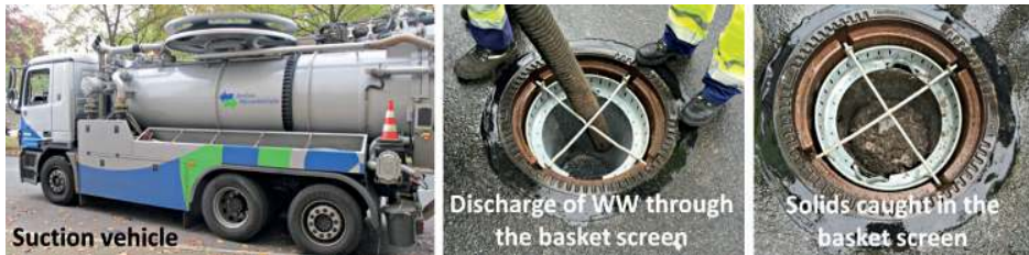
Fig. 6. From left to right: Suction vehicle, wastewater being discharged into the basket screen, basket screen retaining the solid
