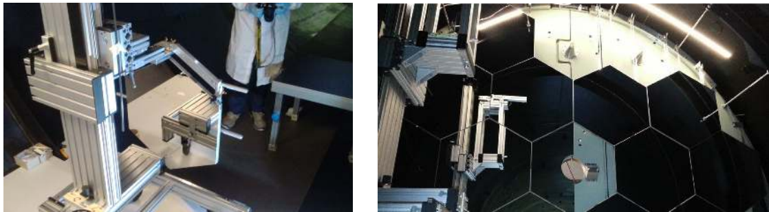
Figure 16. Left: installation tool with a hexagonal mirror ready to be mounted. Right: mirror mosaic close to completion (only two hexagonal mirrors on the top right are missing; the installing tool is visible on the left).
