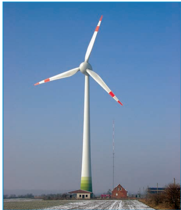
figure 3. Largest wind turbine (currently): Enercon E-112 with a rotor diameter of 112 m and a nominal power of 4.5 MW. (Courtesy: Enercon GmbH.)
