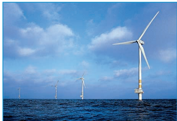
figure 5. Utgrunden off-shore wind farm, consisting of seven 1.5-MW wind turbines erected for the Swedish coast. (Courtesy: GE Wind Energy.)
