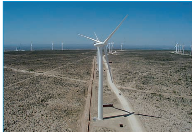
figure 4. King Mountain Wind Range, consisting of 214 1.3-MW wind turbines in Upton County, West Texas. (Courtesy: Bonus Energy Systems A/S.)
