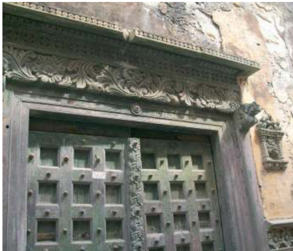
Fig. 1. 'Zanzibari' door, Mozambique Island. Photograph by L. J. K. Bonate.
