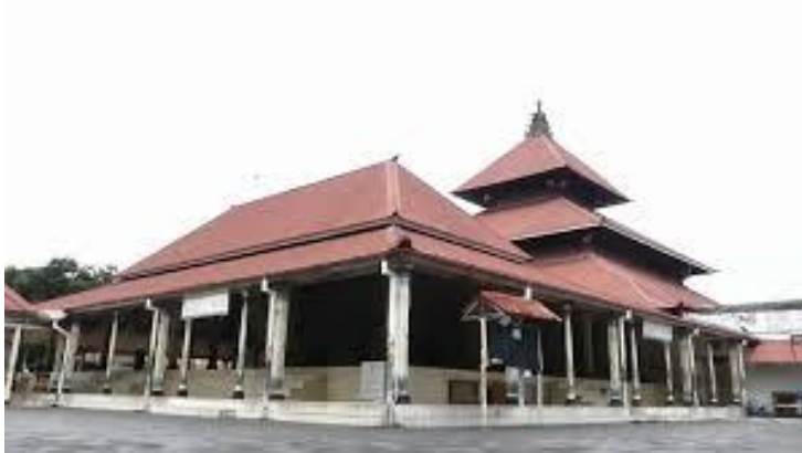
Picture 2. The roof of the Gedhe Kauman mosque is arranged/graded
