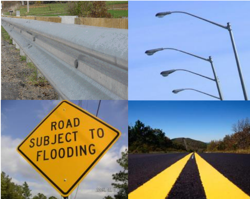
Figure 1. Guardrail, Lighting, Pavement Marking, and Sign Assets (clockwise from top left)
