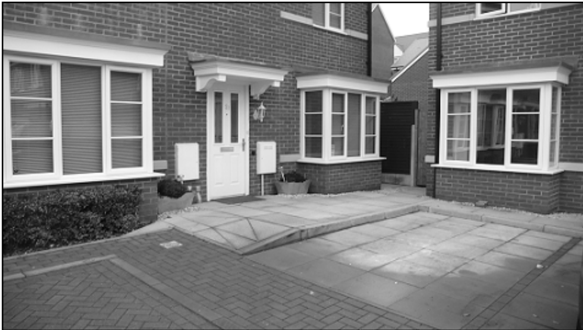
Figure 2: Poor allocation of car parking spaces
