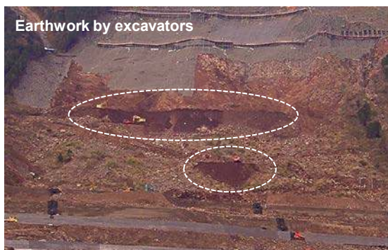
Fig. 12. The areas introducing differential phase after the earthwork due to the wind-driven soil erosion indicated by white dash circles.
