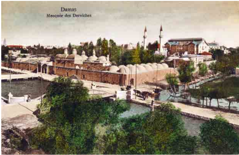
FIGURE 9.5 The Takiyya al-Sulaymaniyya and the Madrasa al-Salimiyya Complex shortly after World War I. The building behind the Takiyya is the Gureba Hospital (from a postcard in the collection of the author).
