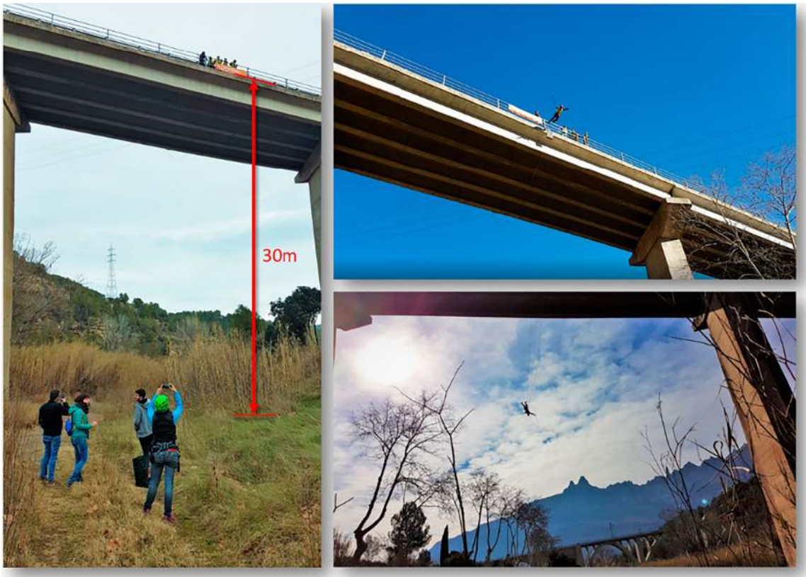
Figure 1. Photographic images of the study settings. General view of the bridge, experimenters, and participants during a jump.
