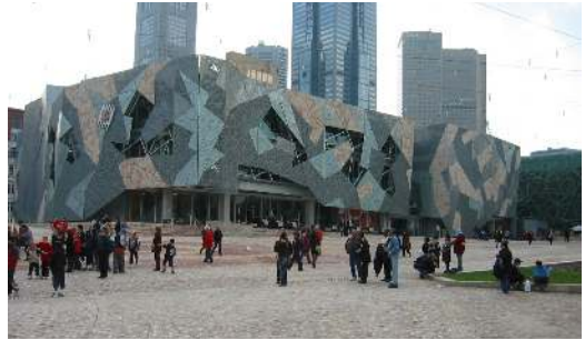
Figure 1. Federation Square, Melbourne, Australia
