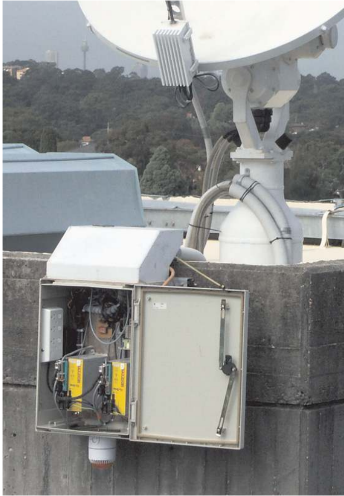
Figure 4.8: Outdoor unit with drive enclosure and pedestal
