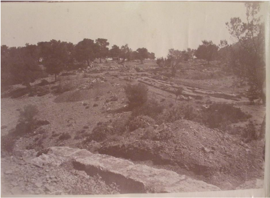
Fig. 40. View of the excavations in 1894 from the south. Note the piles of soil left alongside the excavated buildings. Photo: LUB.
