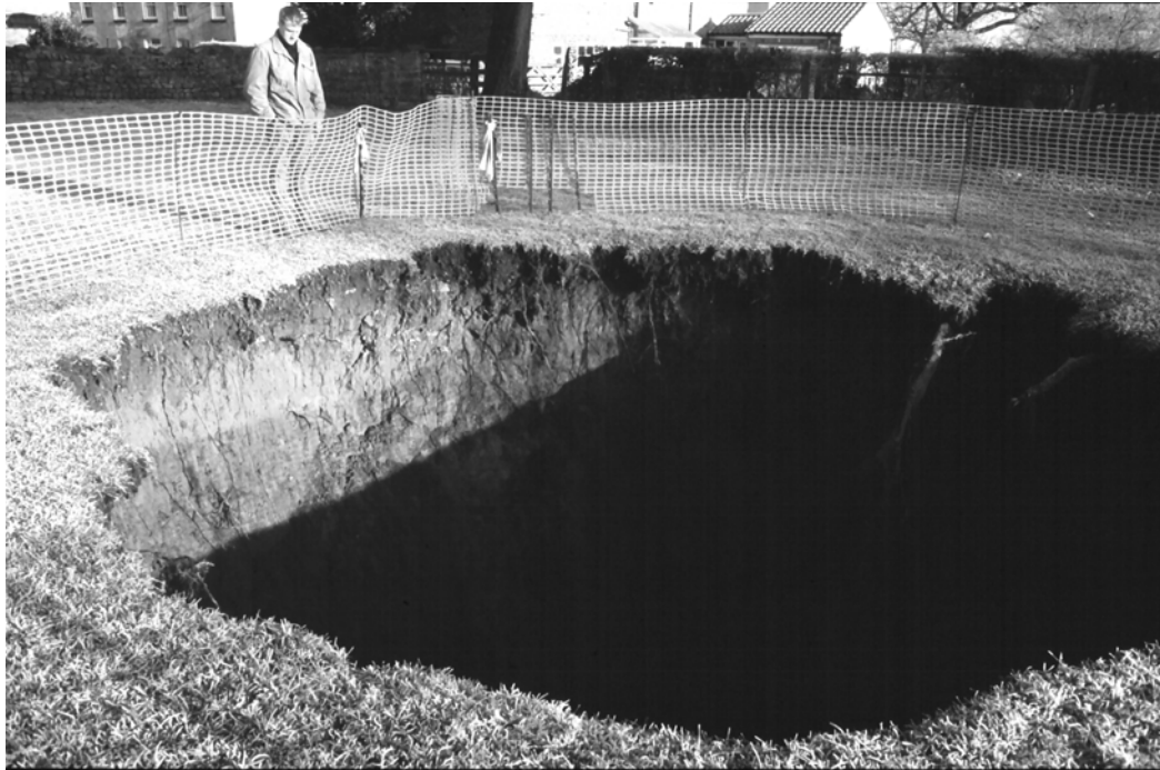
Fig. 7. Sinkhole formed by the dissolution of Permian gypsum in the village of Sutton Howgrave [SE 3246 7928] near Ripon, North Yorkshire. The hole started to collapse in December 2000, the photograph was taken on February 14 th 2001 when the hole was 5-6 m in diameter and 11m deep with water at a depth of 8m. Photo A H Cooper, copyright NERC.
