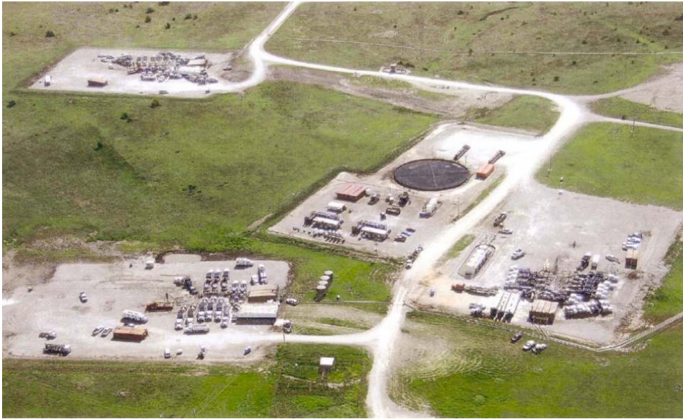
FIGURE 7.0: Barnett Shale Recycling Facility with 2 NOMAD evaporators, with three hydraulic fracturing operations surrounding the facility.
