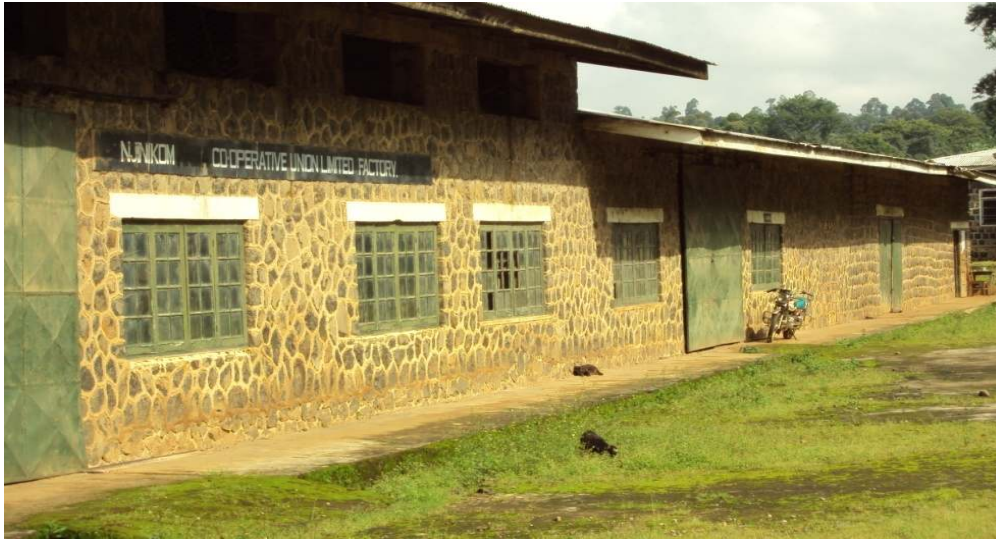
Photo 8.7 The partial view of the building of the Cooperative Union which also houses a coffee mill.
