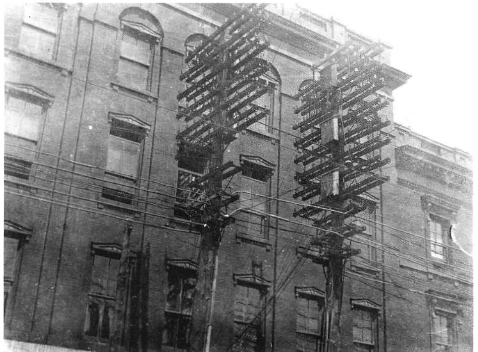
Figure 2: The Wired City. Poles in front of Bell Canada central office, Kingston, Ontario, 1903.
