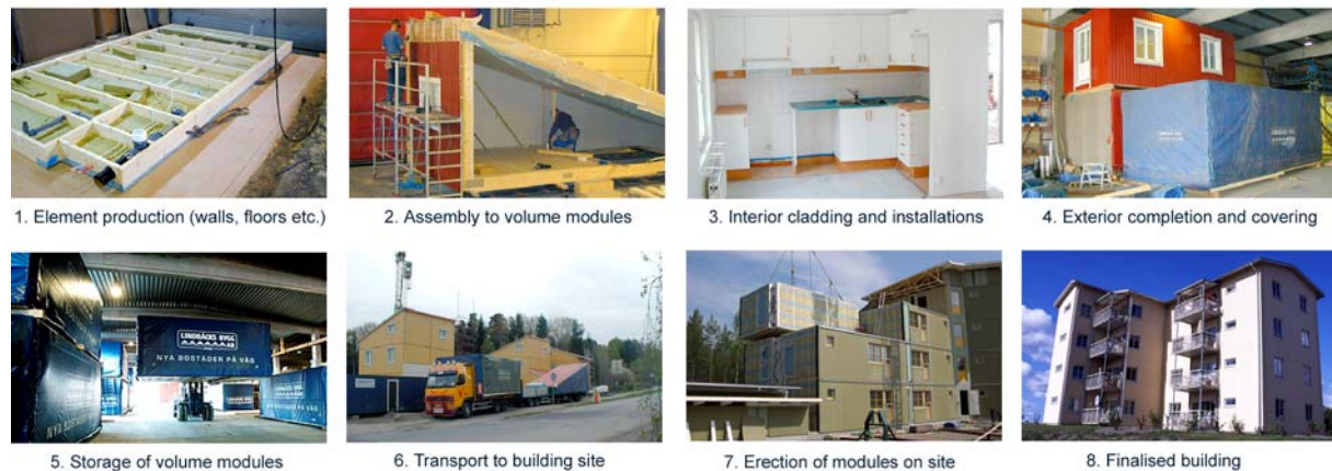
Figure 2. Timber volume prefabrication.
