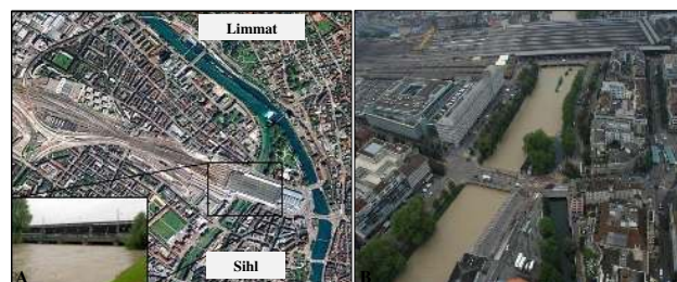
Figure 2. Sihl River flowing beneath Zurich main train station before the confluence with the Limmat River: (a) from Google Maps; in the inset, the situation in August 2005 during a flood event, source: A. Senn (WSL). (b) Sihl River flowing underneath the Zurich main train station in August 2005 (discharge: 280 m 3 s -1 ), source: Office of Waste, Water, Energy and Air, Zürich (M. Oplatka).
