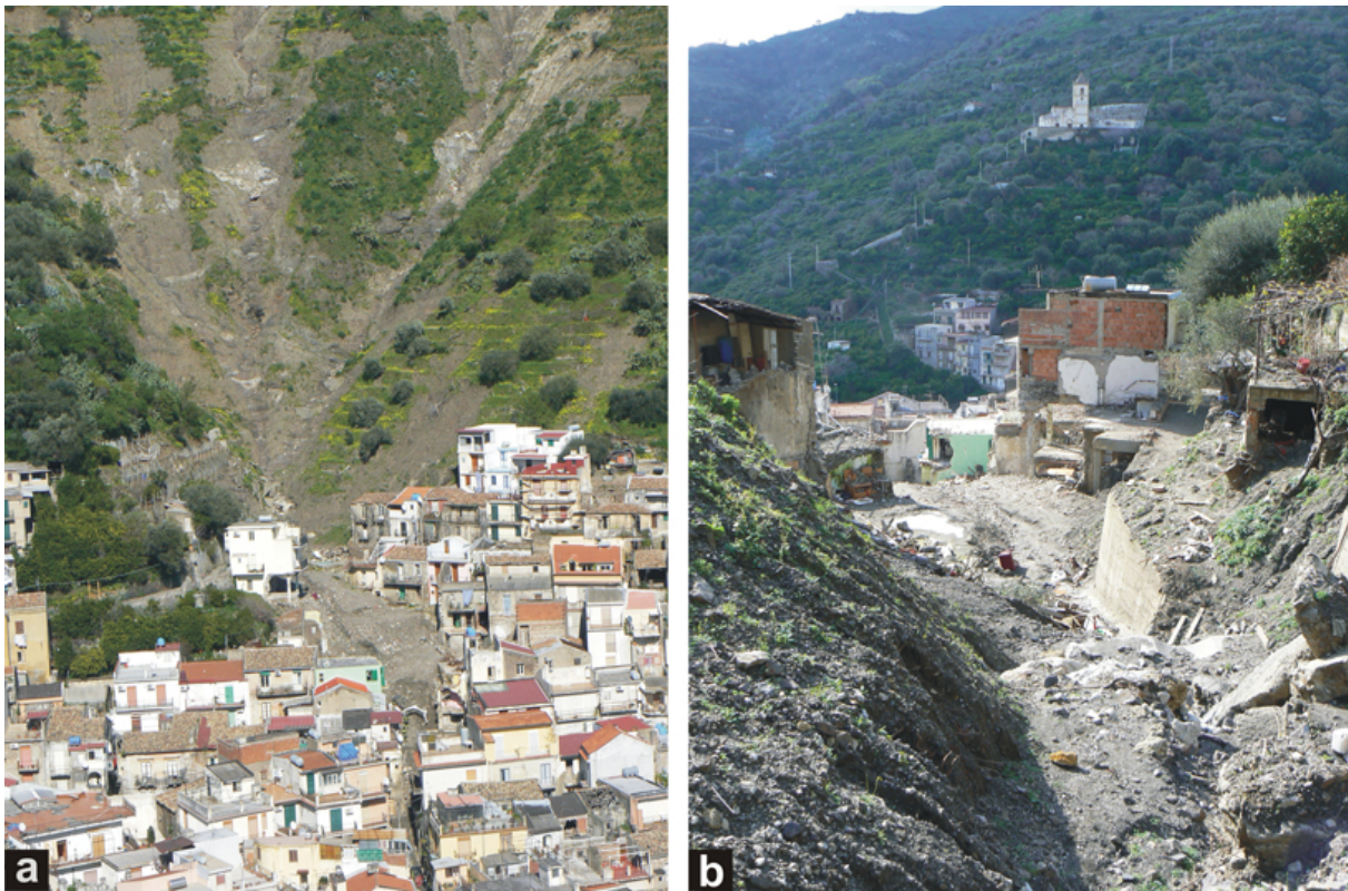
Fig. 2. Examples of some shallow landslides triggered by October 1st 2009 rainfall event in Giampileri village: (a) front view; (b) downslope view.
