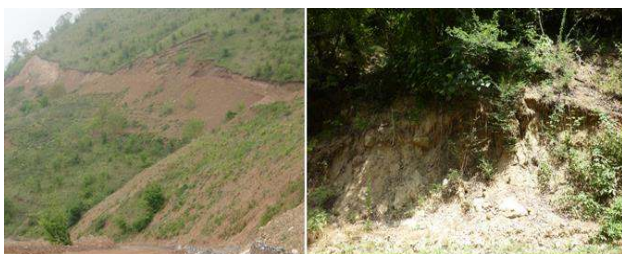
Figure 2. Photos of Landslide in Study area
