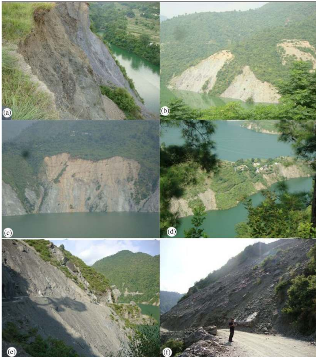
Figure 5. (a, b and c) reflects the landslides due to the reservoir induced side slope saturation, (d) refers to the settlements situated (at risk) around the rim of reservoir, (e and f) show the consequence of unplanned road construction.
