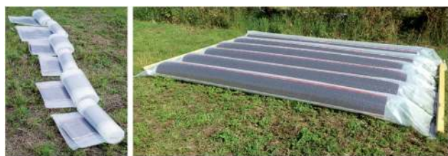
Fig. 4 Ground-based onshore solar cell installation with the rolled-up tubes prior to blow-up (left) and the final setup of six 3.4 m solar cell modules (right).
