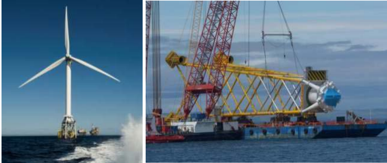
Figure 5-7. Repower 5-MW turbine installed on jacket substructure (left, Talisman Energy, NREL/PIX 17883) and load-out to Beatrice Field (right, Talisman Energy, NREL/PIX 17884)
