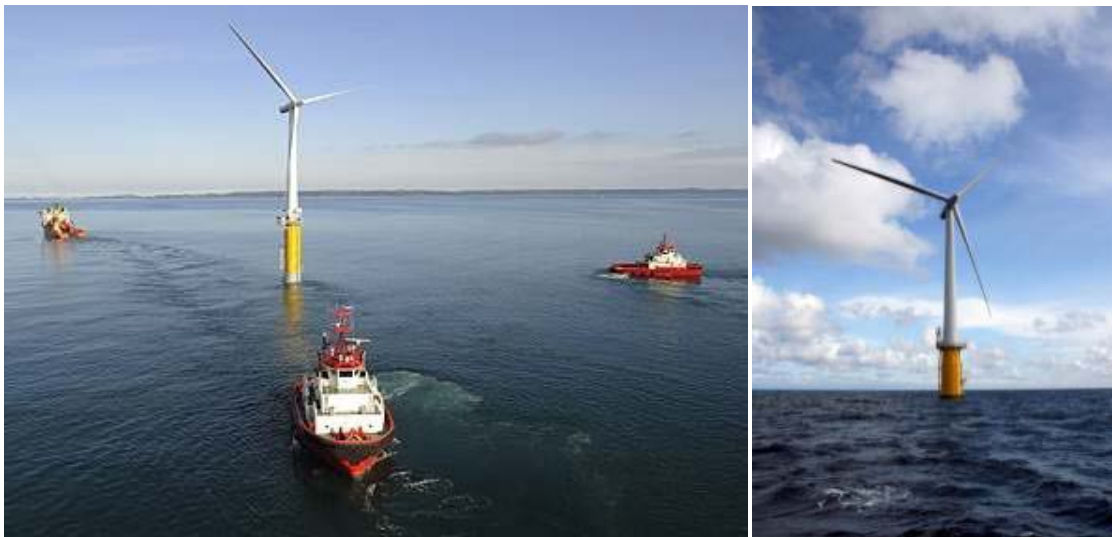
Figure 5-9. First operating deepwater floating wind turbine: Statoil Hywind 2.3-MW prototype during load-out (left) and installed on station (right) (Photos courtesy of Statoil)
