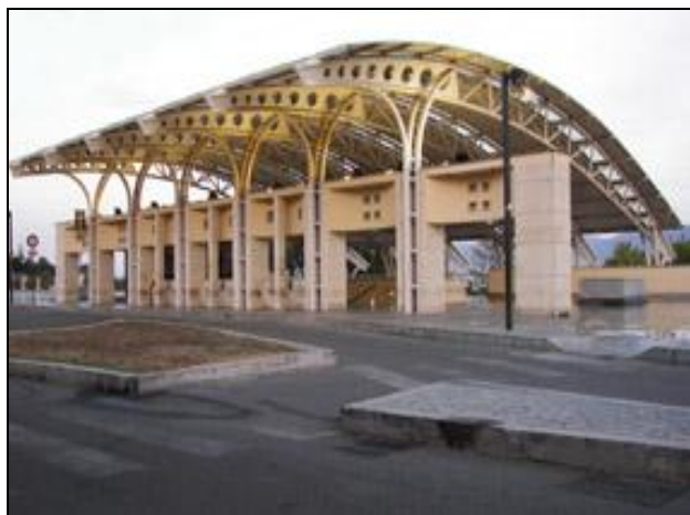
Fig.2: Another view of the covering
