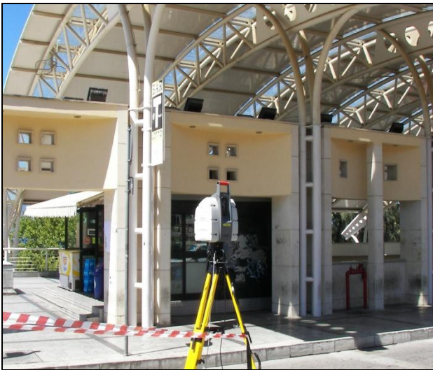
Fig.27: Portion of pillar, object of testing
