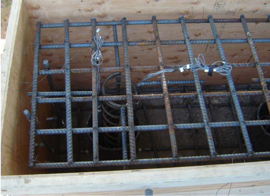
Figure 3-13 Photograph of Pile Cap 1 reinforcing.
