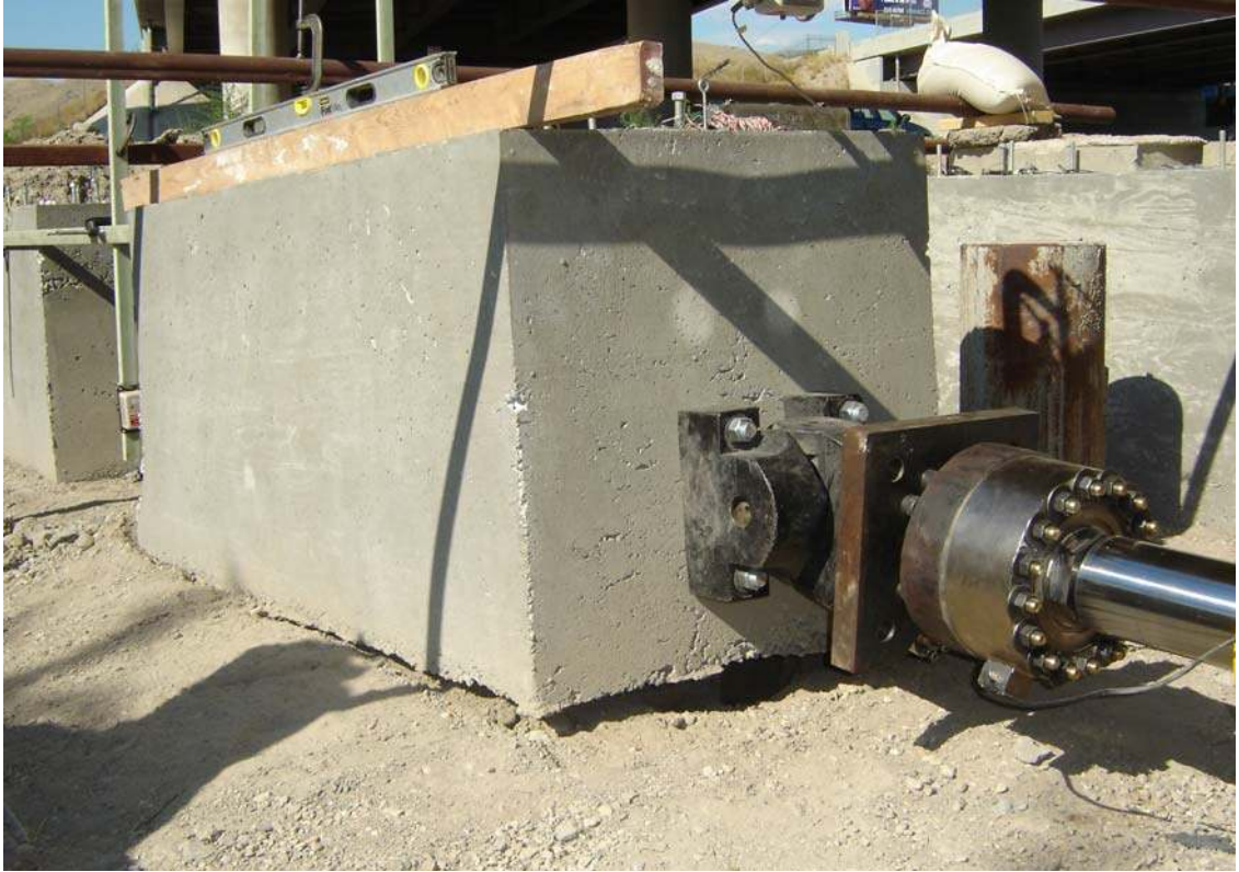
Figure 5-7 Photograph of Test Cap 1 at failure.
