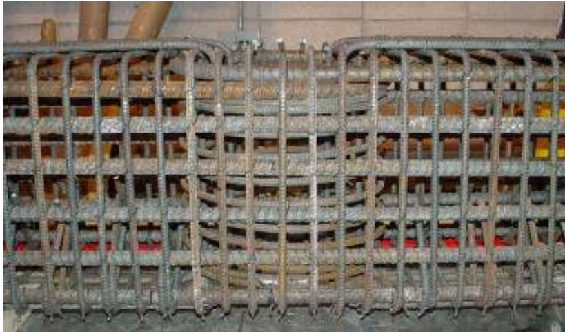
Figure 2-4 Reinforcing cage for pile cap Model 4 Montana State University.
