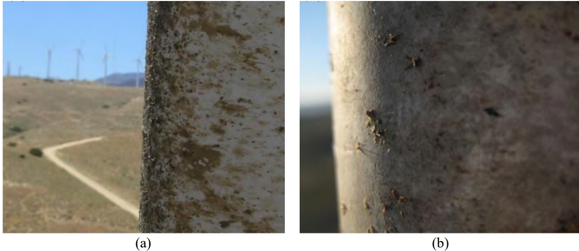
Figure 6 Images of insect roughness on leading edges. (a) Heavy insect roughness from Spruce [43, 44] and (b) minimal insect accumulation from Ehrmann [42]
