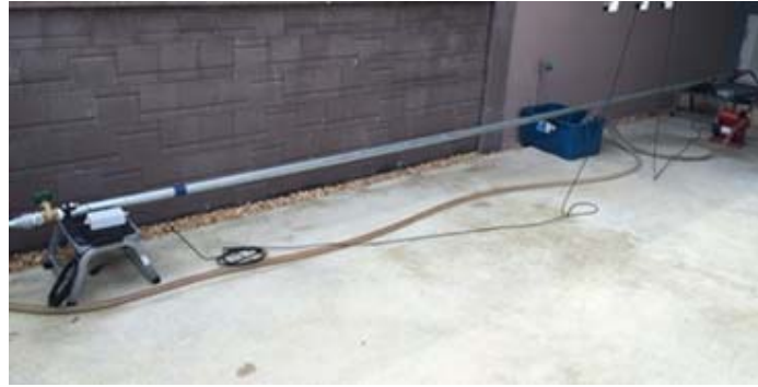
Fig. 3. Pipeline leak detection and localization experimental set up
