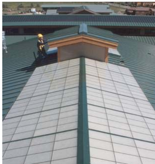
Figure 3-5 Translucent skylights in the roof of the BigHorn warehouse
