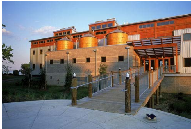
Figure 2-4 North elevation of the Philip Merrill Environmental Center
