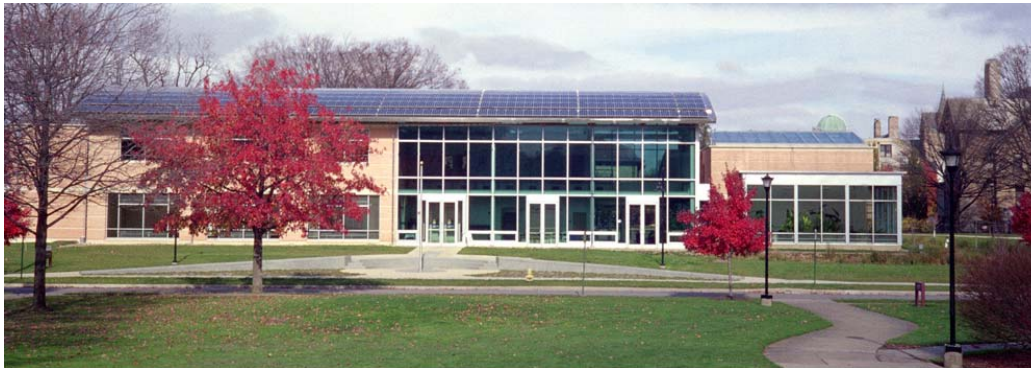
Figure 2-1 South elevation of Oberlin showing roof-mounted PV array
