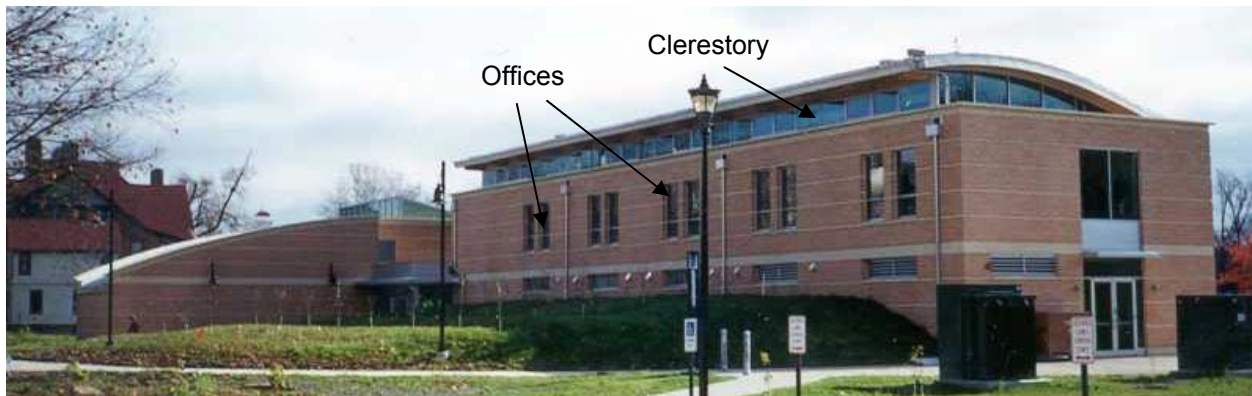
Figure 3-10 Oberlin north facade
