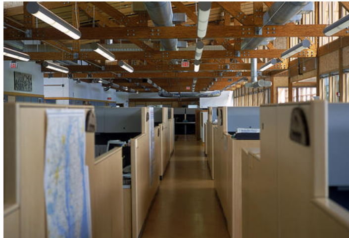
Figure 3-15 CBF second-floor ceiling, beams, and ducts
