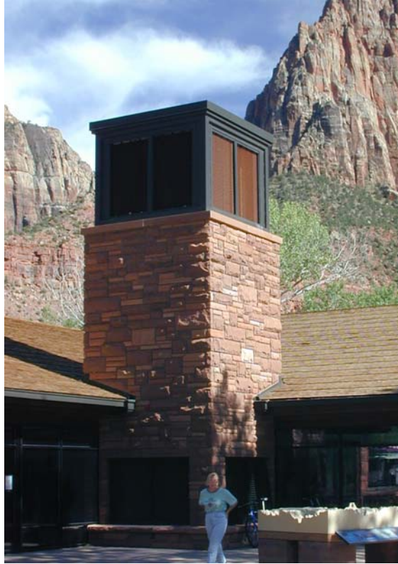
Figure 3-29 Natural downdraft cooltowers—exterior view
