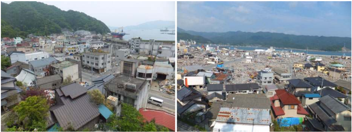
Figure 4 Damage from the tsunami inundation of Kamaishi city with a maximum runup height of 11.7 m (1/6/2011) and of Ofunato city with a maximum runup height of 10.9 m (1/6/2011)
