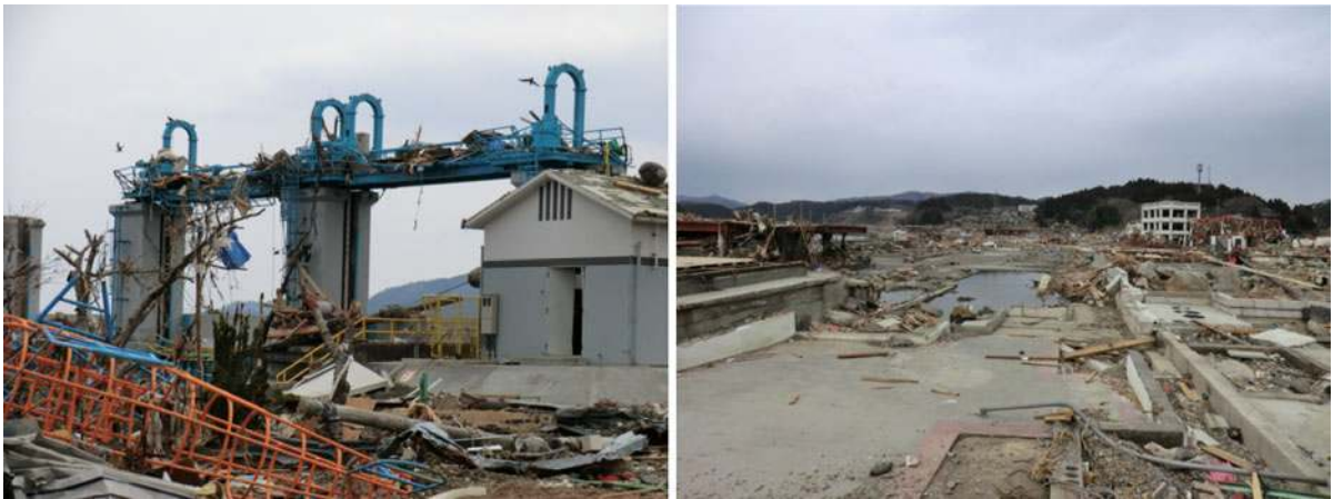
Figure 11 The damaged tsunami gate in Minami-Sanriku town and the town's condition after the tsunami (25/3/2011)
