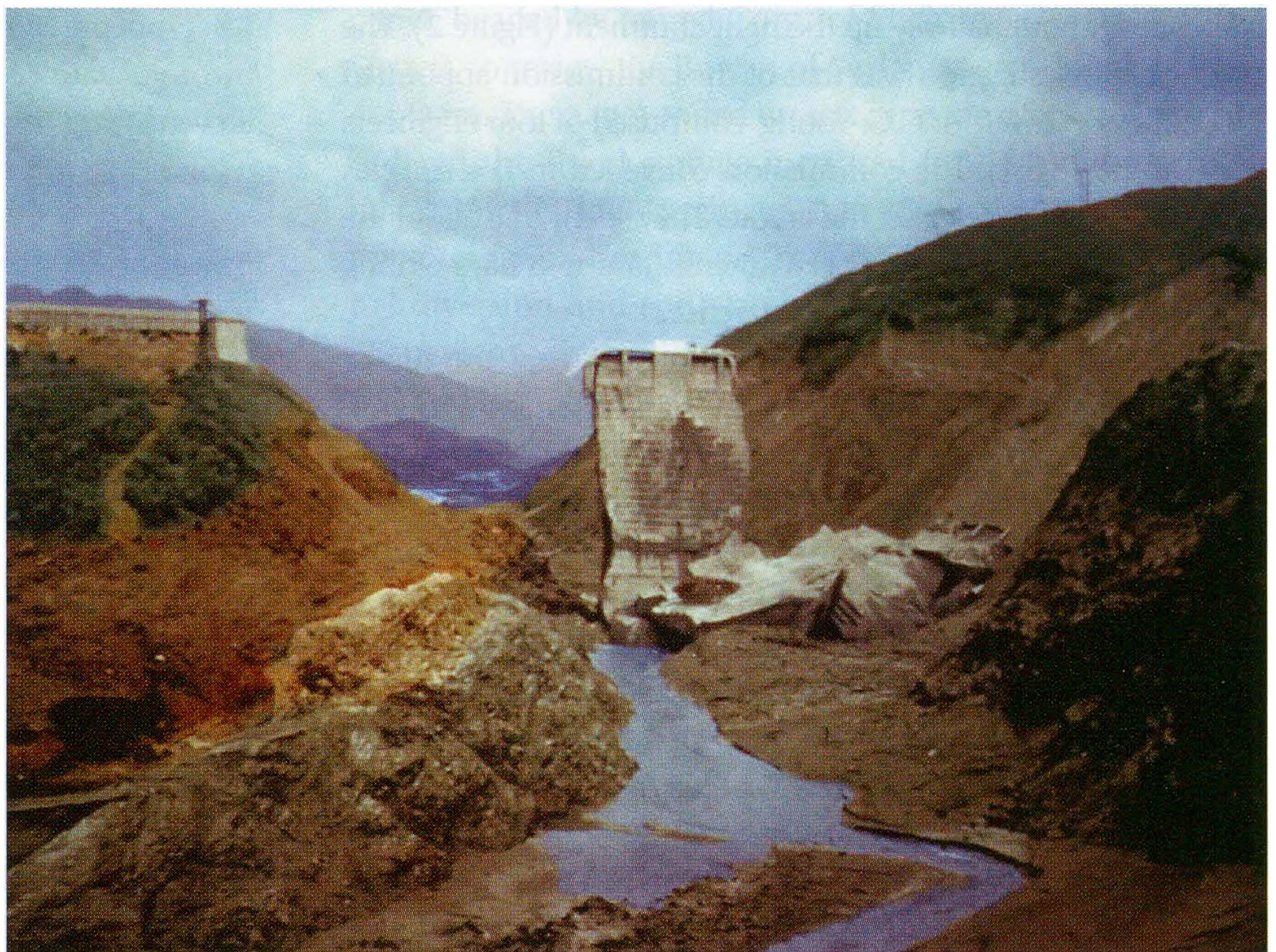
Figure 2. Ground view looking upstream at remains of the St. Francis Dam after its untimely failure in March 1928. Note the dramatic fault contrast between the Vasquez conglomerate at extreme left with the silvery Pelona Schist. The San Francisquito fault pierced the dam's right abutment and was blamed for the dam's collapse (C.H. Lee Collection, U.C. Water Resources Center Archives, Berkeley, colorized by P. Horton).
