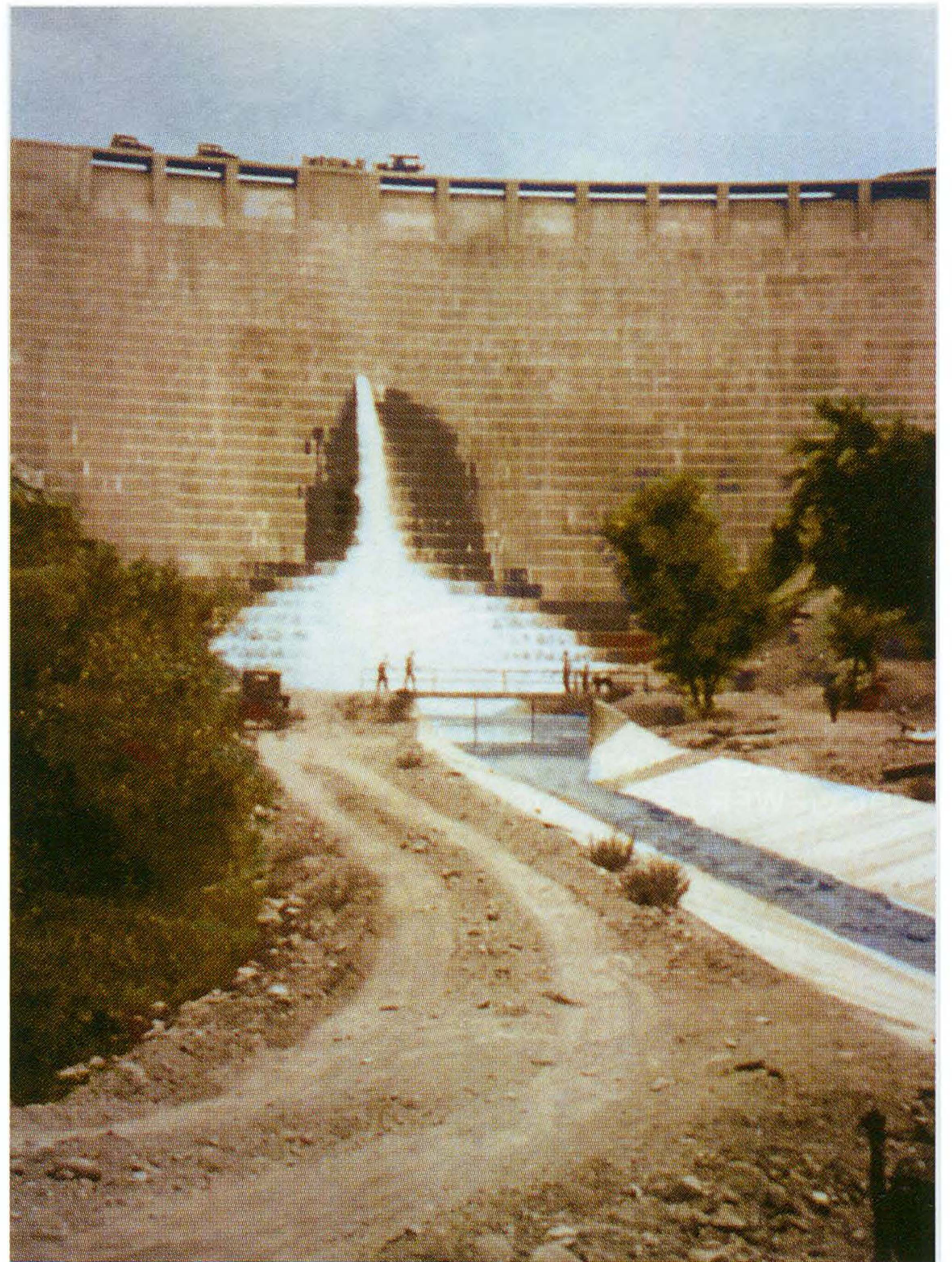
Figure 1. St. Francis Dam was a curved concrete gravity arch structure 209 feet high, constructed between April 1924 and May 1926 (W.L. Huber Collection, U.C. Water Resources Center Archives, Berkeley, colorized by P. Horton).
