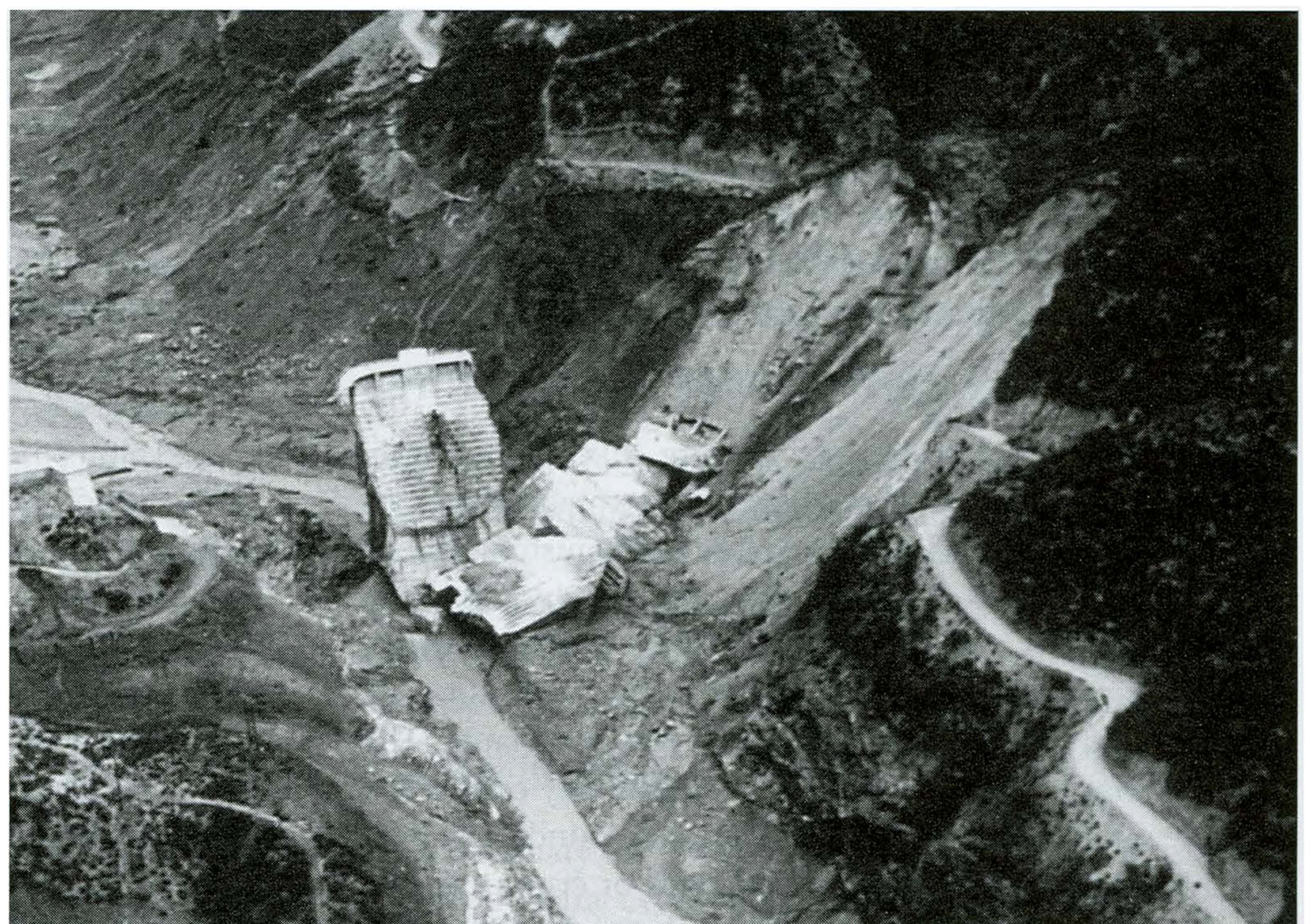
Figure 4. Aerial oblique view of the St. Francis Dam failure taken the following morning, looking upstream. The left abutment landslide is clearly visible, extending almost 200 feet above the reservoir pool elevation (Spense Aerial Photo Collection, UCLA Geography Department).
