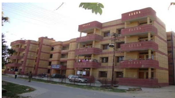
Figure 1. Case study building in Allahabad, India.
