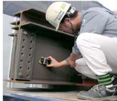
FIG 6: Attaching RFID tag on steel members for progress management (Chin et al. 2008)
